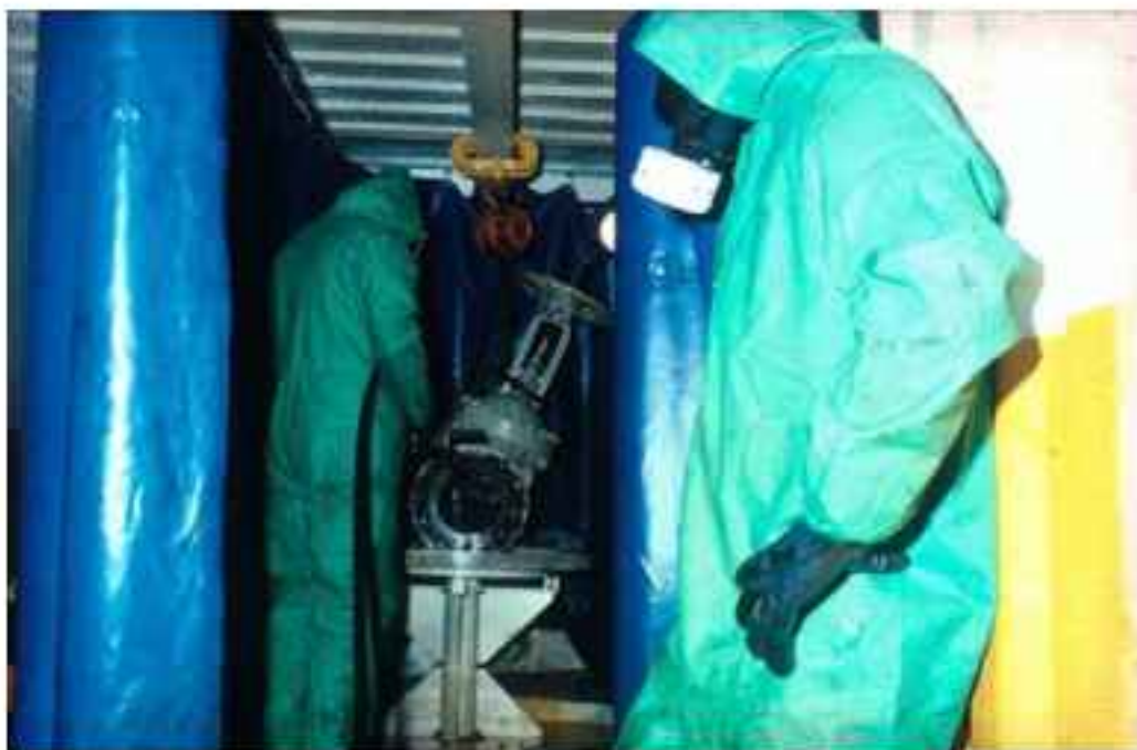
FIG. 50. Workers wearing personal protective equipment decontaminating a valve inside an on-site facility (Courtesy: HPA-RPD, UK)
