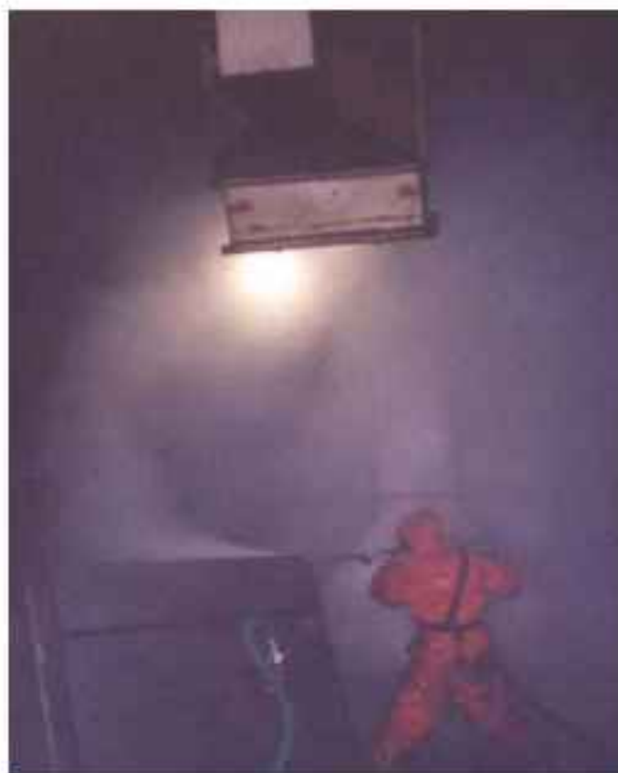
FIG. 54. Worker using a HPWJ lance (overhead extractor removes airborne contamination) (Courtesy: Atomic Energy Commission of Syria)
