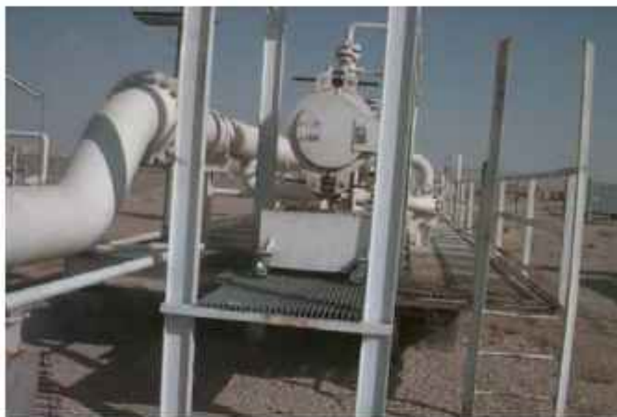
FIG. 14. Pipeline pig trap (courtesy: Atomic Energy Commission of Syria)
