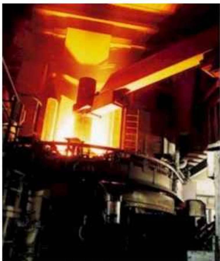
FIG. 57. Melting facility for NORM contaminated materials
