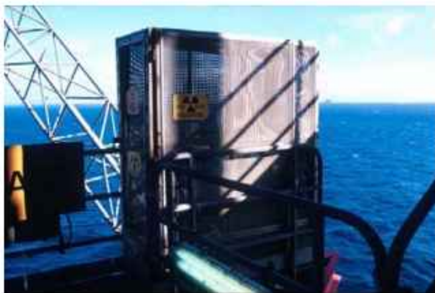
FIG. 25. Store for radioactive sources (Courtesy: HPA-RPD, UK)
