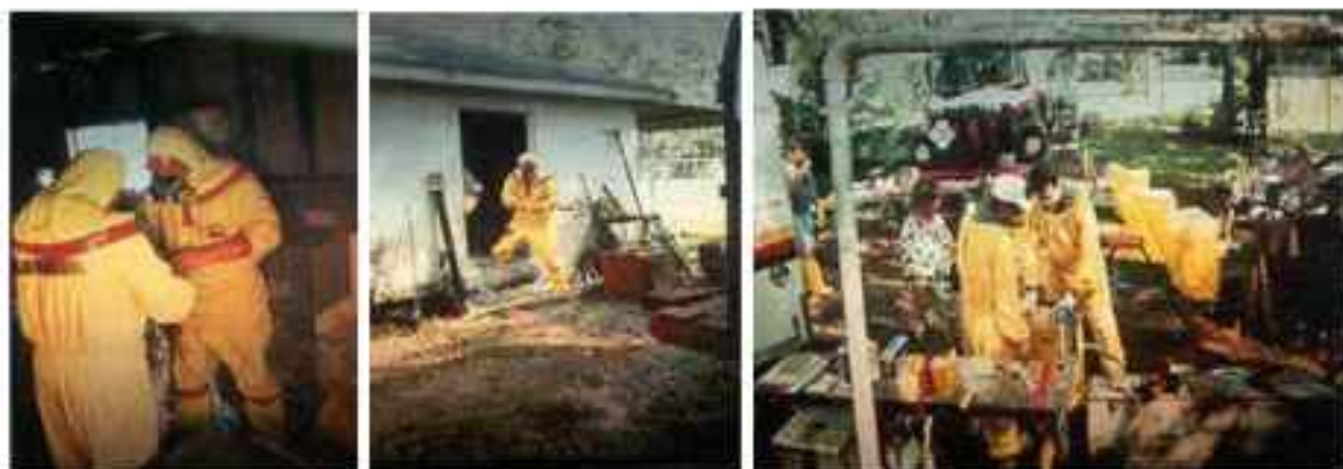
FIG. 87. Retrieving (left), handling (centre) and packaging (right) of ruptured source
