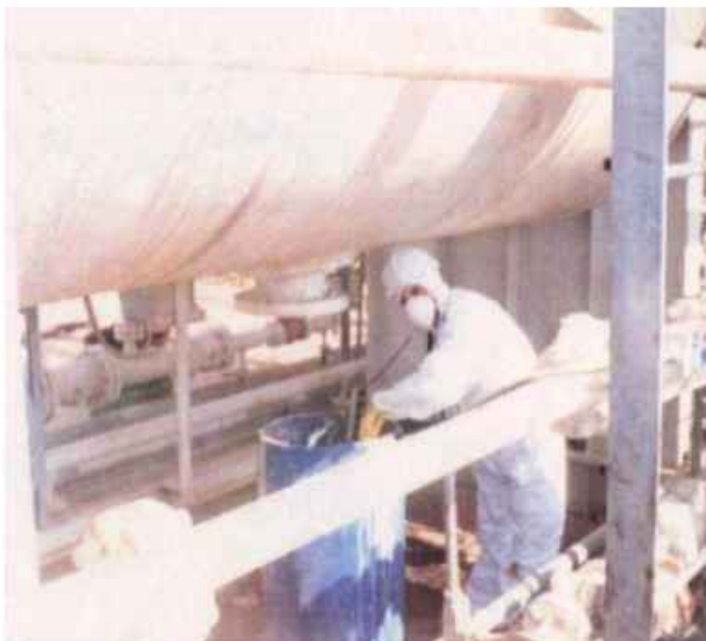
FIG. 52. Removal of bulk sludge from a vessel (Courtesy: Atomic Energy Commission of Syria)
